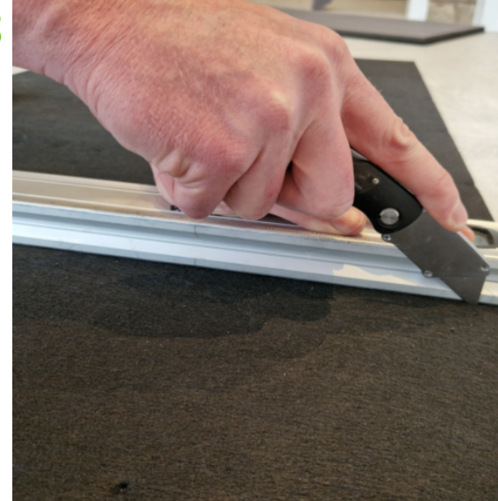
Cut felt with a utility knife
