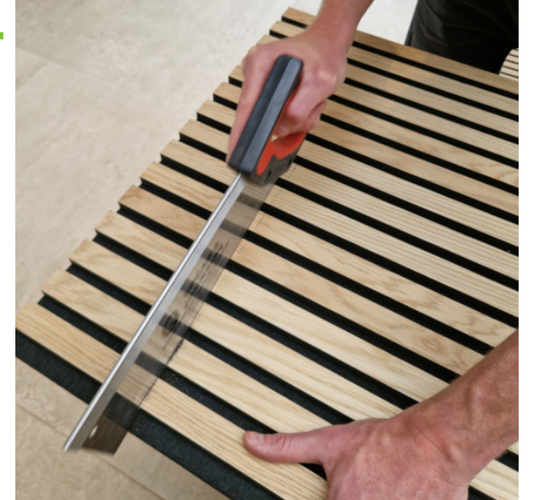
Cut with a fine-tooth hand saw
